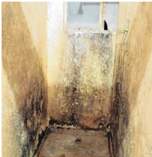
PRIMITIVE: A shower area in the old hospital.
